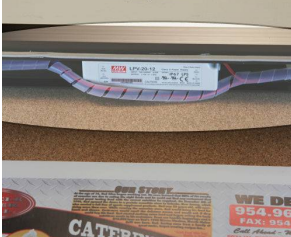
Ballast/Transformer concealed inside Display Case
