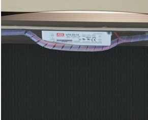
Ballast/Transformer concealed inside Display Case
