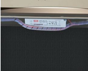
Ballast/Transformer concealed inside Display Case
