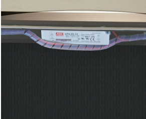
Ballast/Transformer concealed inside Display Case
