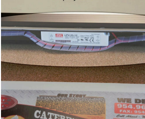
Ballast/Transformer concealed inside Display Case
