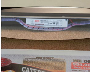
Ballast/Transformer concealed inside Display Case
