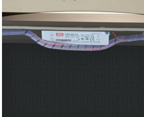
Ballast/Transformer concealed inside Display Case
