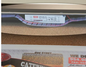
Ballast/Transformer concealed inside Display Case
