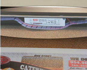
Ballast/Transformer concealed inside Display Case
