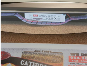
Ballast/Transformer concealed inside Display Case
