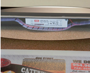
Ballast/Transformer concealed inside Display Case
