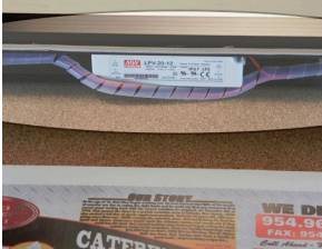
Ballast/Transformer concealed inside Display Case
