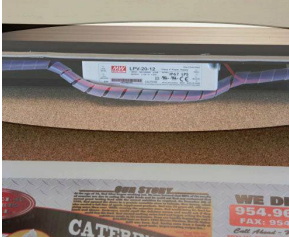
Ballast/Transformer concealed inside Display Case
